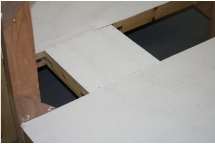
Another of these has a length of baton screwed to the side, slightly offset
